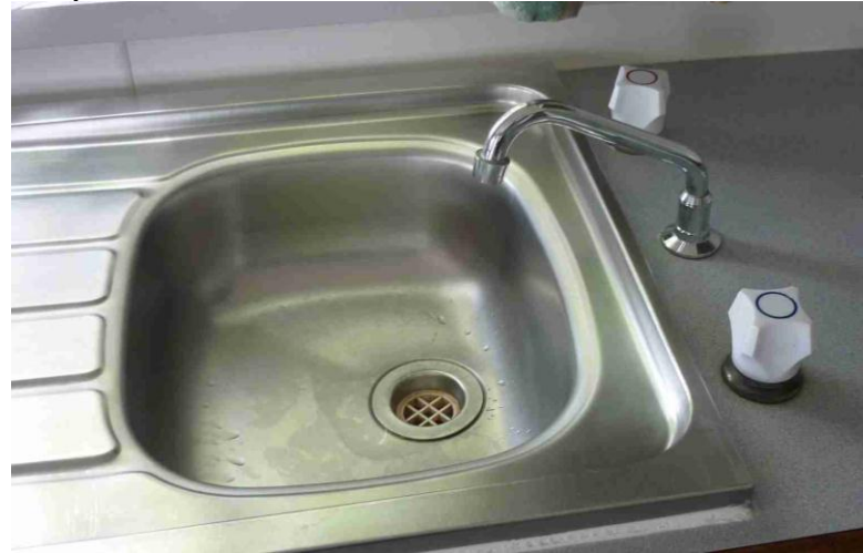
Figure 5. Example of a Kitchenette Tap at Wodonga Caravan and Cabin Park
